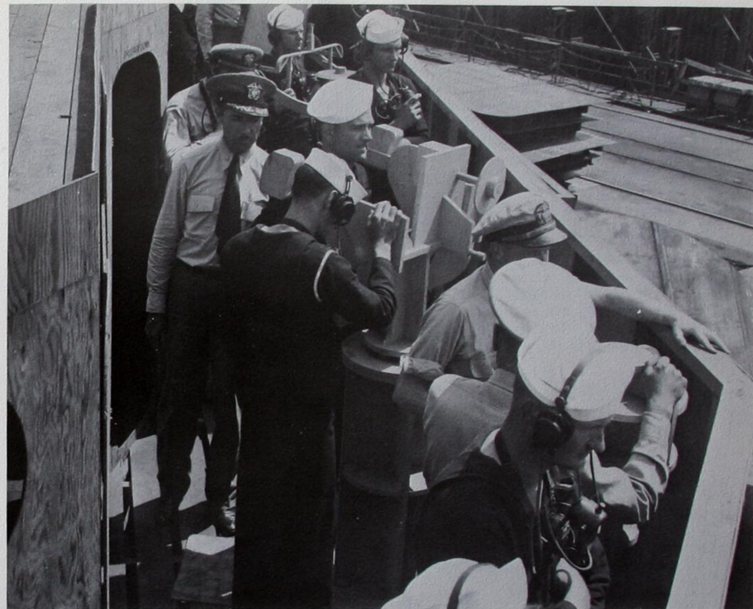
DE HAVEN's first crew practices on mockup of ship which was then under construction.
